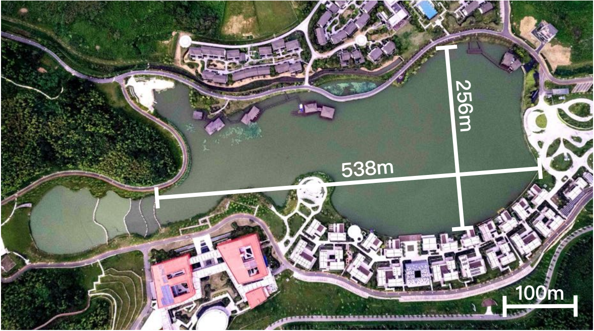
Figure 3.7: Overhead View of Experimental Site, Huzhou, Zhejiang
